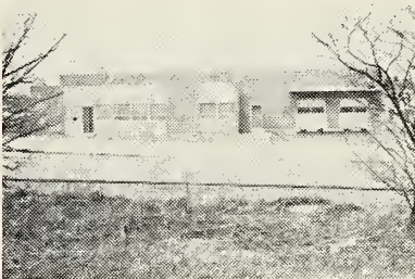
EXTERIOR OF PLANT located at 1210 Glendale-Milford Road.
